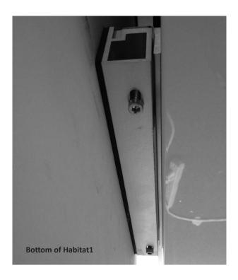
22 Secure bottom bracket with the two 50mm long cap head hardware provided from the bottom side of the bracket.
