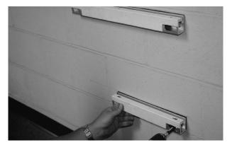
18 Screw bottom bracket to wall using screws. Make sure screws are tight and bracket is mounted securely to wall.
