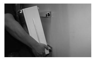
17 Connect AC cable provided to back panel of Habitat1. Lift cabinet to wall and lower onto brackets.
