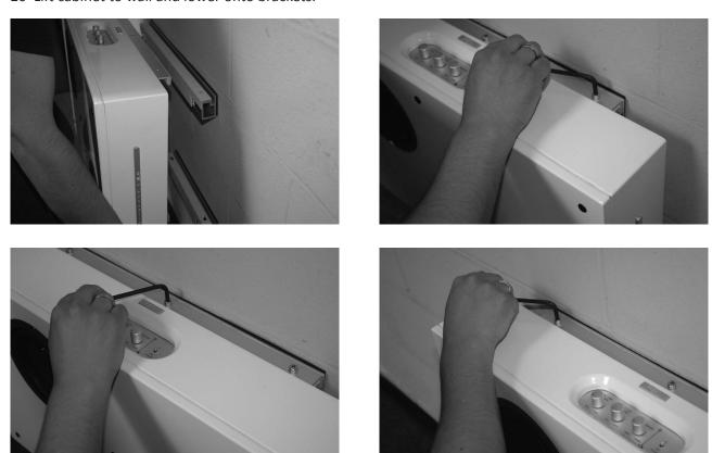
21 The fit will be snug. Draw the cabinet into place using the three 13.5mm long cap head top mounting hardware. Tighten the three provided screws 1/2 turn at a time starting with one side and rotating through each one. Tighten the three provided screws 1/2 turn at a time starting with one side and rotating through each one. Using this method will take several passes to get the screws tight. You will notice that with each pass the Habitat1 is evenly pulled into the bracket.
