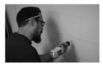
8 Drill hole for anchors using the drill / driver and 5/16 drill bit.
